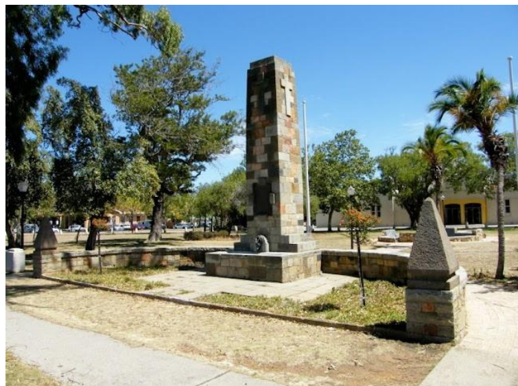
Scenes from the Walmer Cenotaph repairs.
